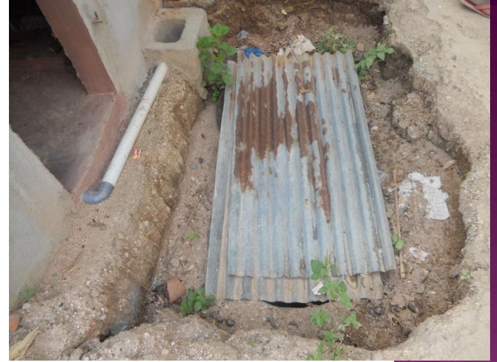
Open septic tanks
