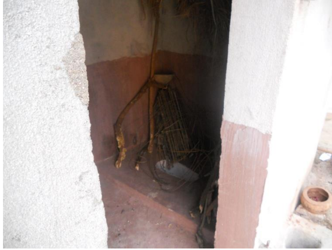
Pucca Toilet used as storeroom
